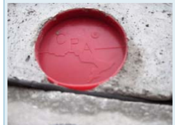
Tank Talk promotes the CPA Product Registration Program and encourages building inspectors to look for this Red Tag or other evidence of compliance
